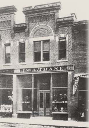
Trane Storefront La Crosse, Wisconsin 1891
